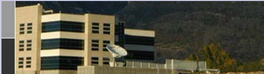
The Atvantage Data Center in Lindon, Utah
