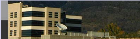
The Atvantage Data Center in Lindon, Utah
